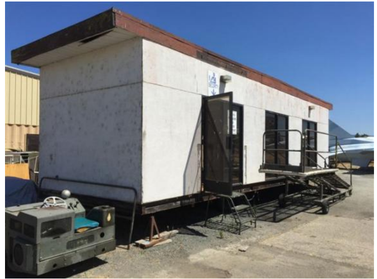
This new PCAM acquisition needs your help. The photo at left shows some of the water damage that needs repairing.
