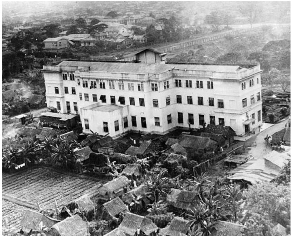
One of the main buildings of the Santo Tomas Dominican College, converted into dormitories for civilian internees. Shanties built by the prisoners are visible in the foreground, with a tilled field at the left. This U.S. Army photo was taken in 1945.
