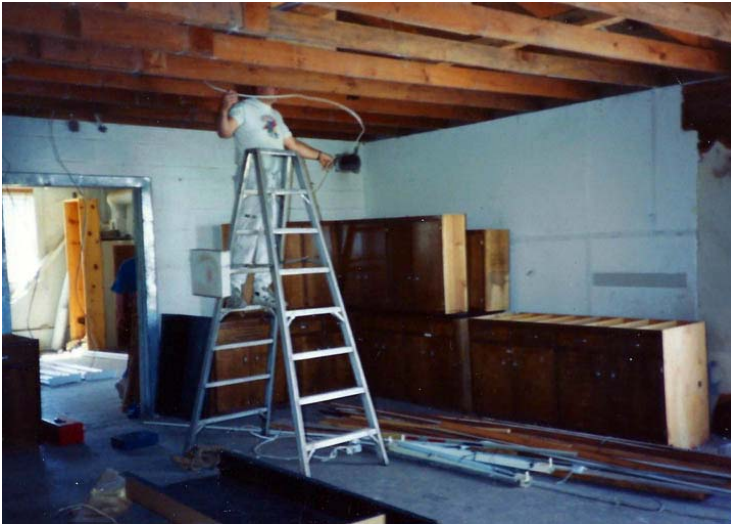
Installing lights in what is now the Gift Shop.
