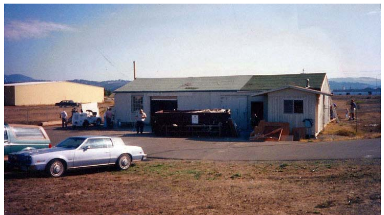
The PCAM building in the early days, under refurbishment and while we were still meeting in the STS control tower. Where are the planes? The fences? The CAP building? All were yet to come.
