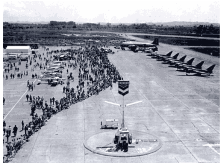
May 1967: Airport Appreciation Day, early forerunner of Wings Over Wine Country Air Show. Courtesy Sonoma County Airport
