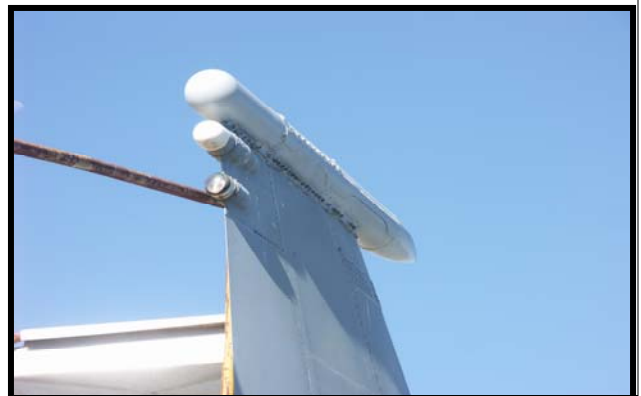
The Damage Repaired (6/21/2011)
