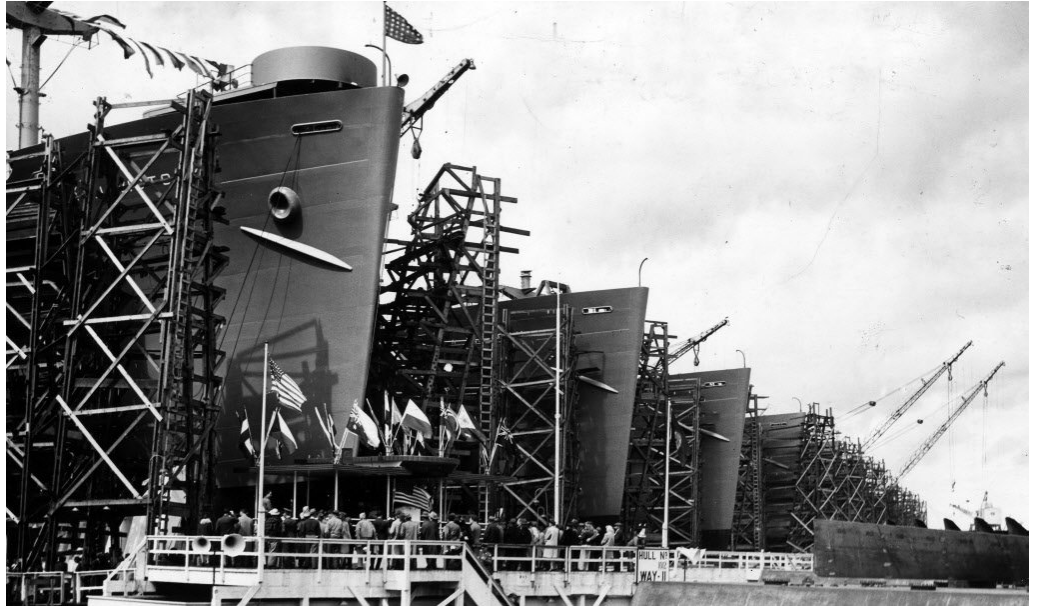
Kaiser revolutionized shipbuilding by first welding together huge sections of ships assembly-line style, then lowering these modules into place with enormous cranes. Kaiser's shipyards in Portland, Oregon (above) and Richmond, California could crank out a Liberty Ship in a few days, a rate unheard of before World War II.
